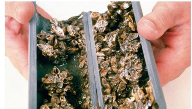
(a) Clogging a pipe
