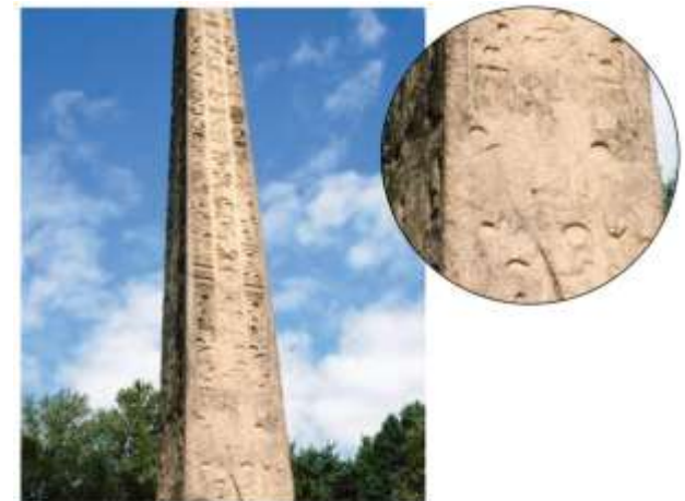
(b) After acid rain damage
